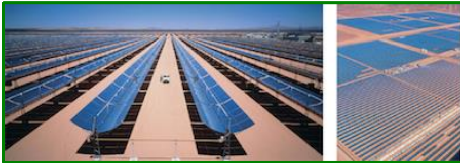
Luz International plant in California . Solar Electricity Energy System (SEGS). Heat synthetic oil to 390 °C. Competitive with PV.
