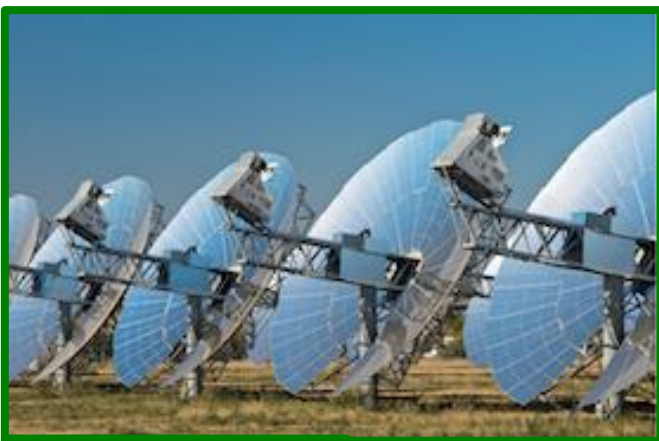
Here is an array of 60 parabolic dishes each with a 25 kW Stirling engine apparatus, which can operate at very high temperatures, up to 1,000 °C, which will result in high efficiency, constructed in Arizona in 2010
